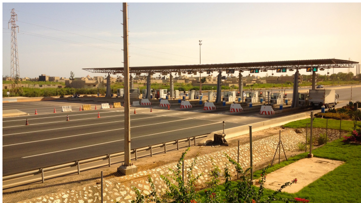
Dakar-Diamniadio toll motorway in Senegal.
